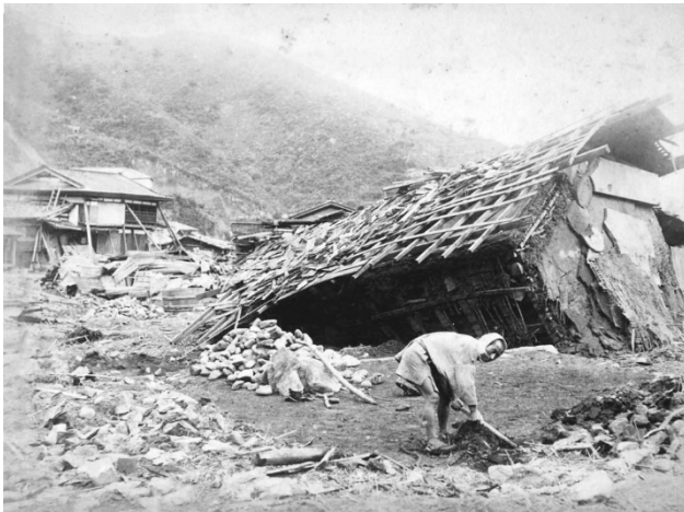
Figure 1.8 Destruction in Kamaishi city, Iwate prefecture due to the Sanriku earthquake (a photo credited by Matsuchi Nakajima, 1850–1915, in Wikimedia Commons).
