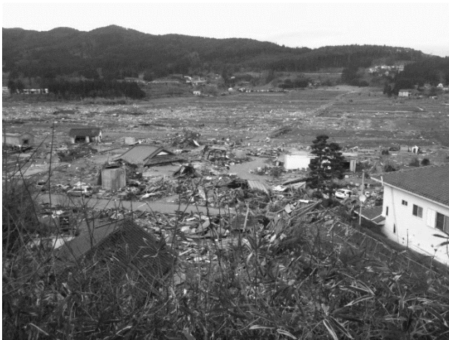
Figure 1.10 The Rikuzentakata, Iwate, after being swept by a tsunami on the Pacific Coast following the Tōhoku earthquake (a photo credited by Mitsukuni Sato, in Wikimedia Commons).
