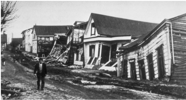
Figure 1.4 Earthquake damage to good quality, wooden-framed houses in Valdivia, Chile, 1960 (a photo credited by Pierre St. Amand, from Wikimedia Commons).
