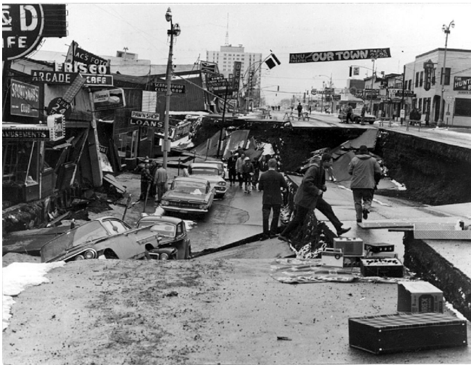
Figure 1.12 Damage to Fourth Avenue in Anchorage, Alaska, caused by the 1964 Alaska earthquake (a photo credited by the U.S. Army, in Wikimedia Commons).
