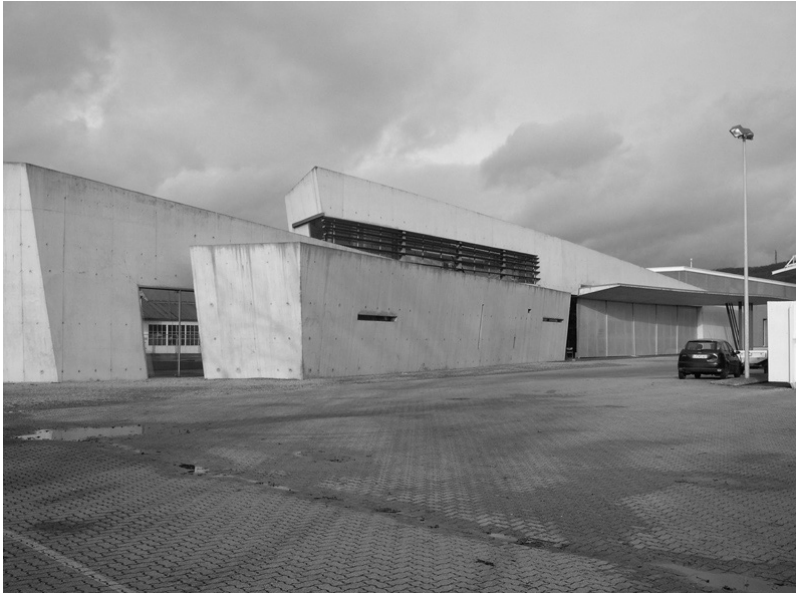
Figure 1-3: Vitra Fire Station
