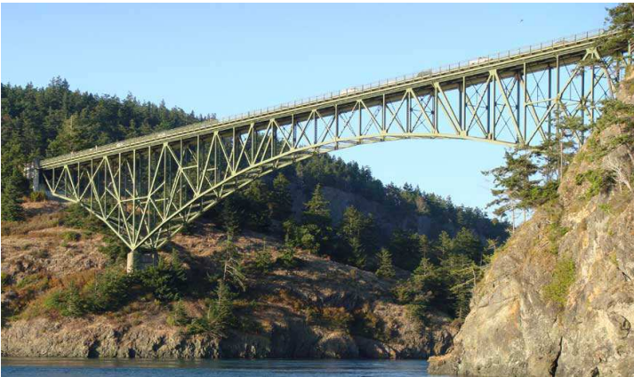
Fig. 3. Road bridge in Seattle, WA, USA
