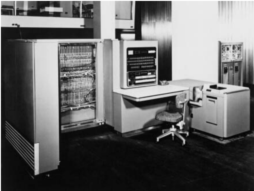
Figure 1-1. IBM 701 Electronic Data Processing Machine
