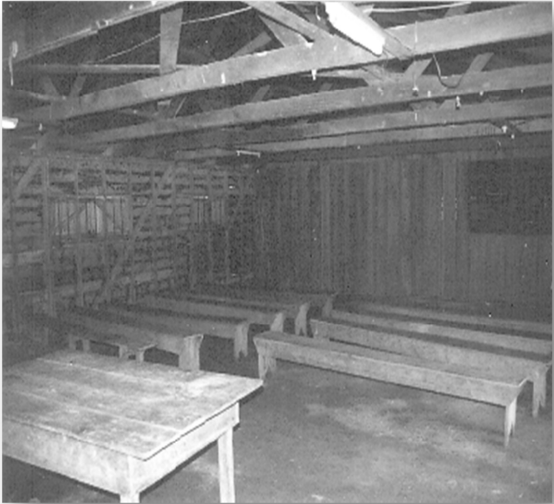
Fig. 1.2. Interior existing hurricane shelter (photo submitted by I. Tait)
