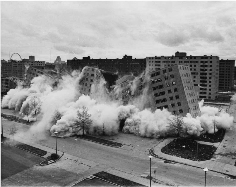
Fig. 1-1 Demolition of Pruitt-Igoe March 16 th 1972 [Source: Wikimedia Commons]
